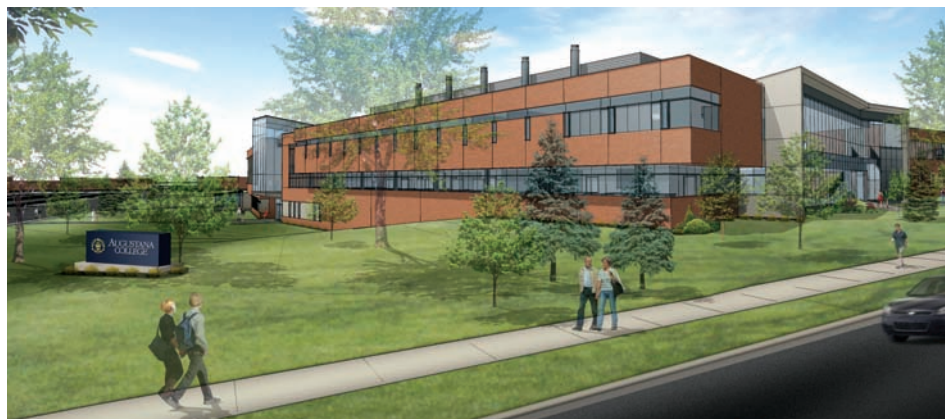
Artist rendering of the New Gilbert Science Complex from 33rd and Summit.
