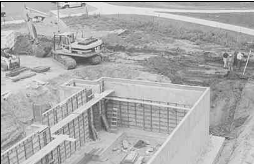
June 8, 2000, the service basement walls of the Fantle Building are complete, as crews begin work on the southwest foundation.
