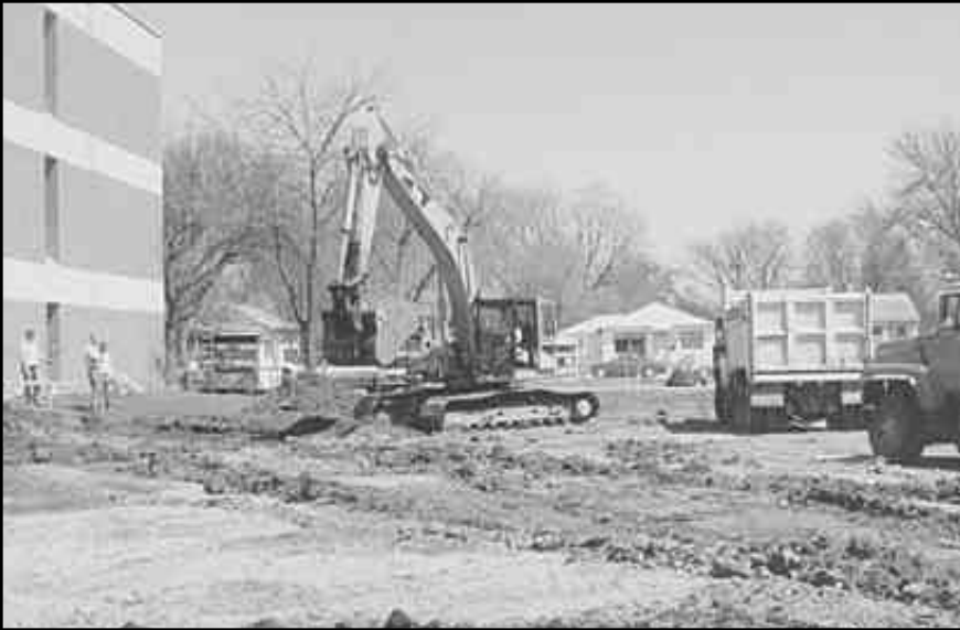
April 25, 2000, Swift Contractors begin work on the Fantle Building for the Center for Western Studies.
