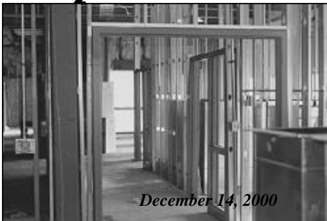
The steel frame for the lobby area is being erected.
