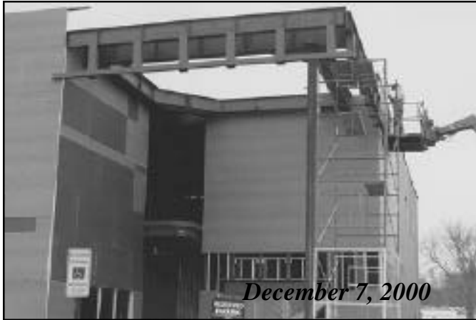
The steel frame for the lobby area is being erected.
